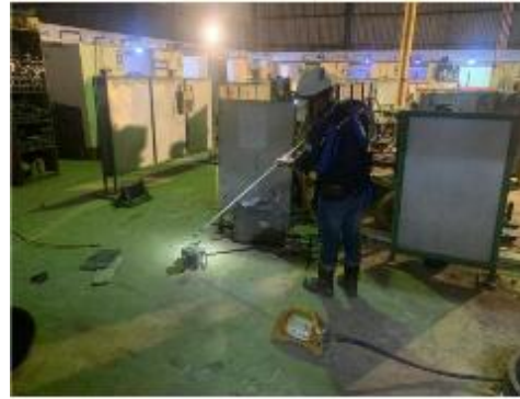
Recovery Ir-192 source in emergency pit
